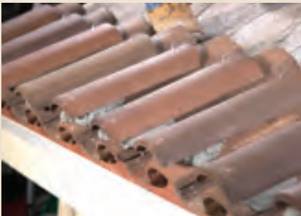
Boosting The Eave
