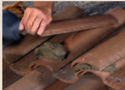
Placing The Mortar*
