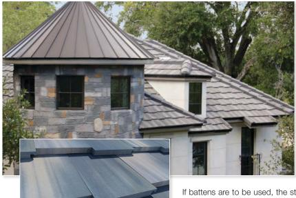
Installing a staggered exposure can seem daunting to an installer that has not done one before. The truth is that it is really quite simple. It just requires planning. The first thing to think about is waste. Remember, that approximately half of the tiles on the roof will have a shorter exposure than the other half. It will be essential to calculate that difference prior to ordering the tile.
