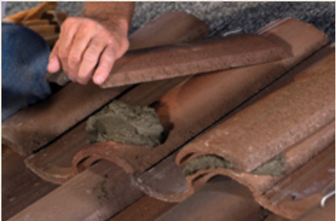
Placing The Mortar
