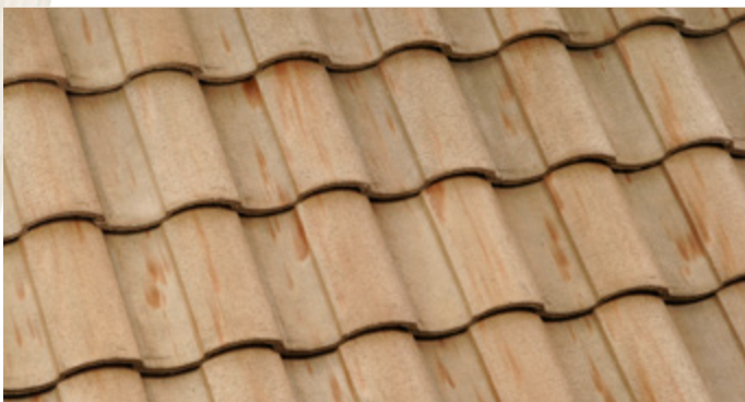
3530 Weathered Adobe - Tan, Rust Streaks
