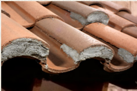
Close-Up of Boosted Eave
