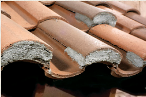
Close-Up of Boosted Eave
