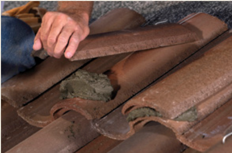
Placing The Mortar
