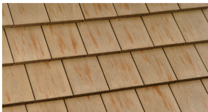
4530 Weathered Adobe - Tan, Rust Streaks
