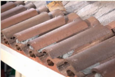
Boosting The Eave
