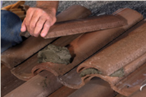
Placing The Mortar
