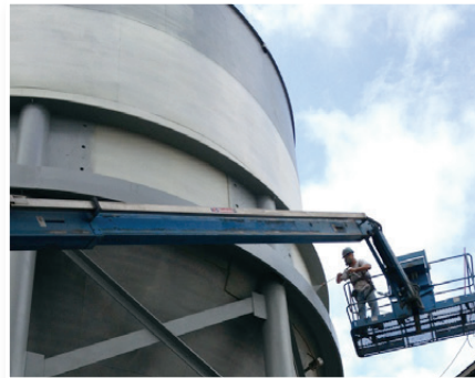
Tank Insulation Coating: Weyerhaeuser paper manufacturer; Savannah, GA
