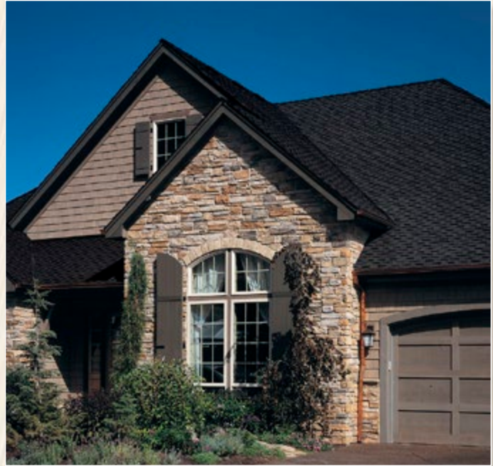
Asphalt Shingle. Temporary, basic roof covering.
