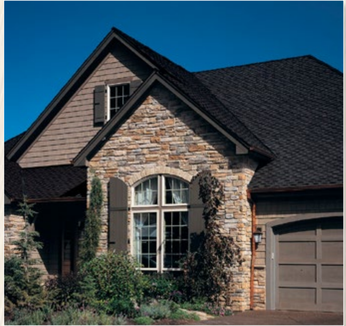
Asphalt Shingle. Temporary, basic roof covering.
