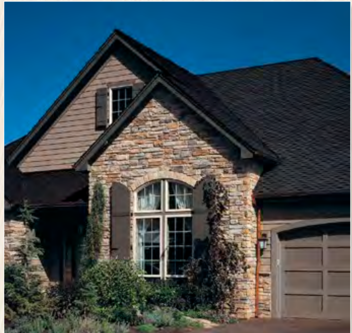
Asphalt Shingle. Temporary, basic roof covering.
