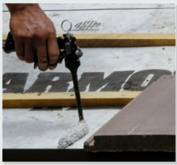
**The Dual Fix Hybrid System** provides the verifiable and proven peace of mind of knowing that the roof system is secure. Whereas with a dual-component tile adhesive installation, it takes post-installation destructive testing or a wind event to determine if the concealed attachment method was mixed properly, installed as prescribed (proper paddy size and placement) or actually exists.
