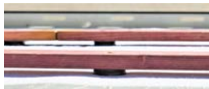
OPTIONAL BATTENS WITH SHIMS, RAISED PADS
