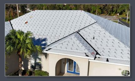
Valor Thermal is comprised of layers of 99% highly polished, scrim reinforced aluminum, thin, insulative fiberglass, and synthetic underlayment. The result? A product that is revolutionizing the roofing market and helping roofers meet new fire and energy codes.
