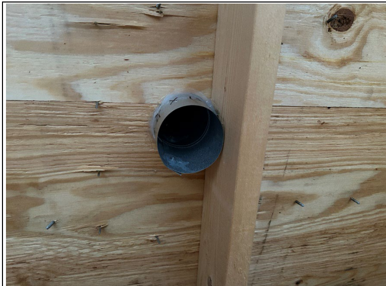
Photo No. 2 Underside Before Testing
