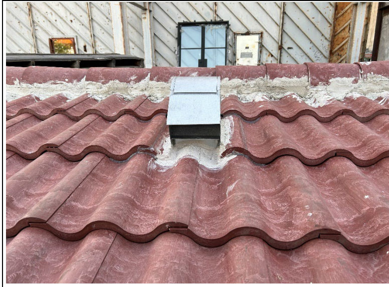
Photo No. 1 Top Side Before Testing
