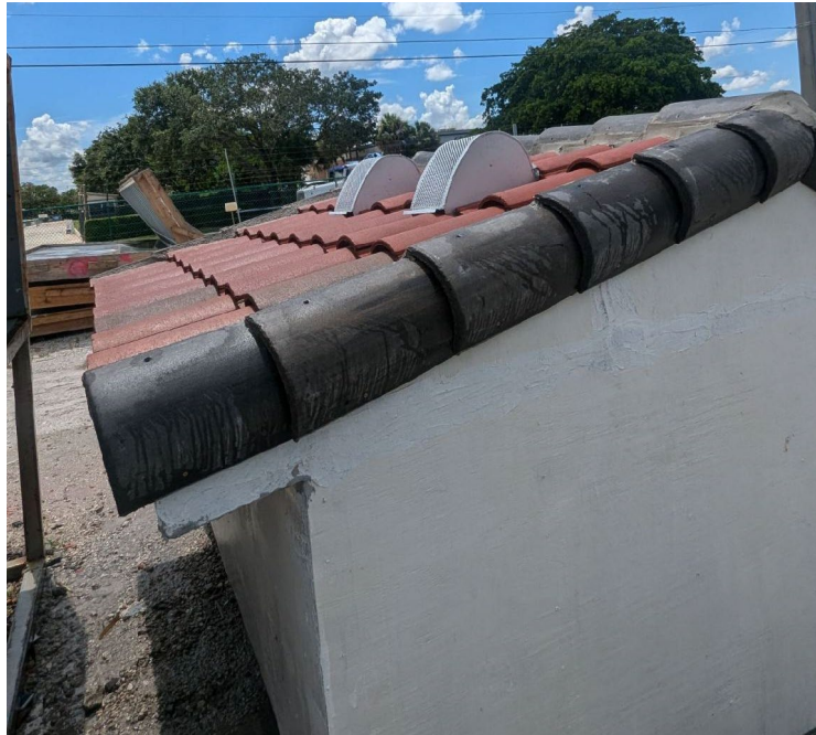
Photo No. 1 Right Side of Deck
