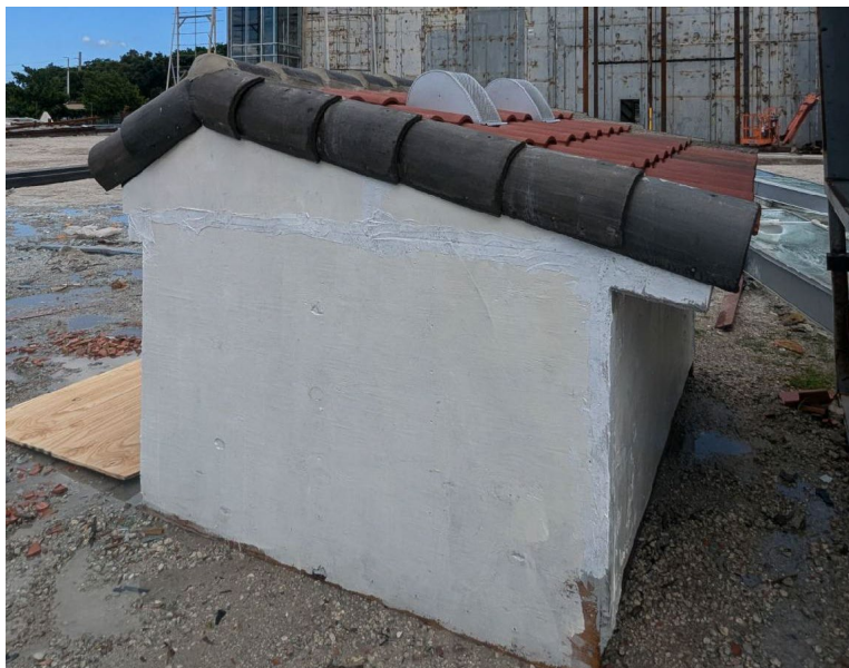
Photo No. 2 Left Side of Deck
