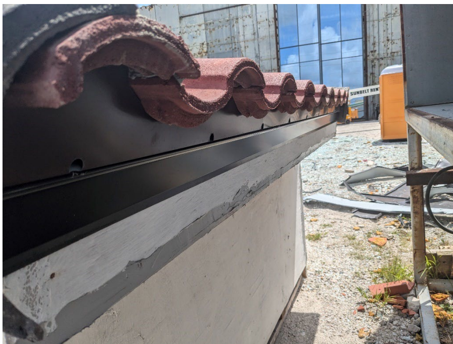
Photo No. 3 Windward Edge of Deck
