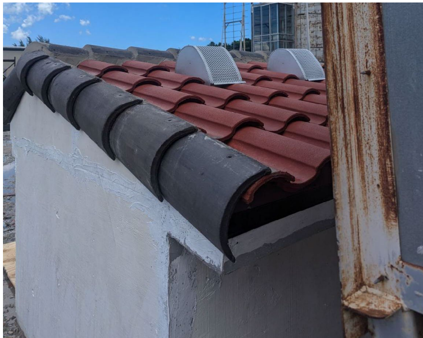
Photo No. 3 Front Side of Deck
