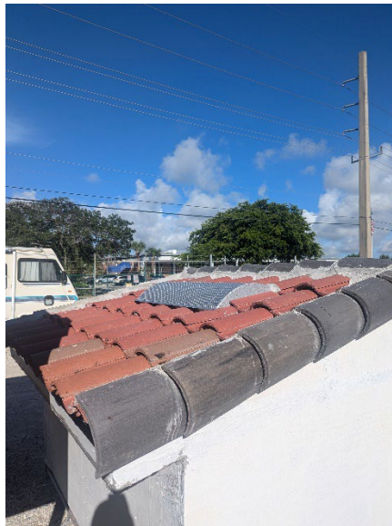
Photo No. 2 Top Side After Testing
